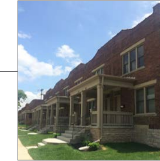
Community Properties of Ohio Renovation A public/private partnership provided a $30 million renovation of 300 project-based Section 8 units (2009).
