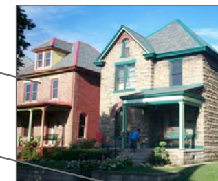
Scattered Site Exterior Home Repair Program Nearly $3 million was raised from private sources to support 70+ exterior home repair grants (up to $20,000 each) to improve roofs, windows, siding, foundations and energy efficiency (2011-2016).
