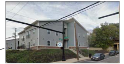
Trolley Park development New residential building with 18 two and three bedroom units.
